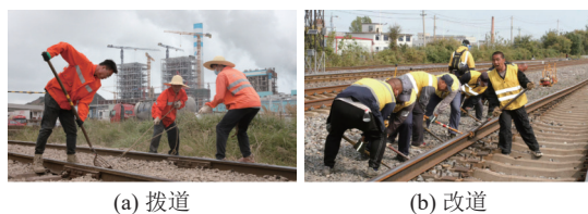
图 29 铁路拨道和改道 Fig.29 Diversion and rerouting of railways
