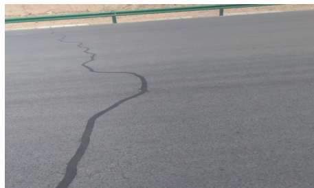
图 30 修补路面裂缝 Fig.30 Repair of pavement cracks
