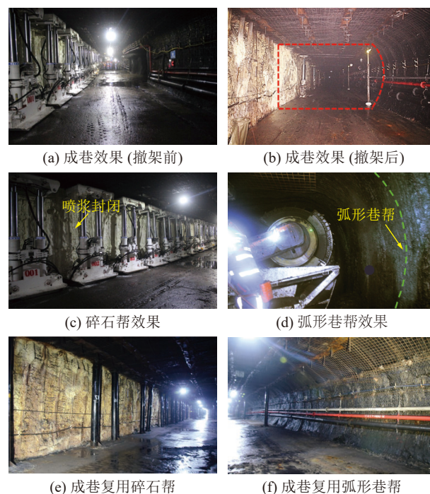
图 19 典型矿井 N00 工法成巷效果 Fig.19 Roadway forming effects of N00 mining method
